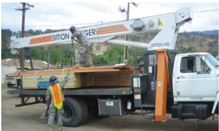
A construction crew delivers rebuilding materials
