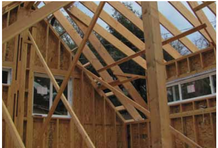
Reconstruction in progress
