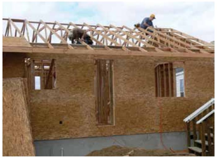
Construction continues on an MDS home
