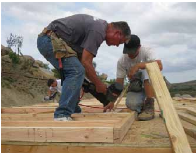
MDS volunteers framing a new home
