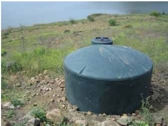
New water tank provides gravity-fed irrigation to restored habitat
