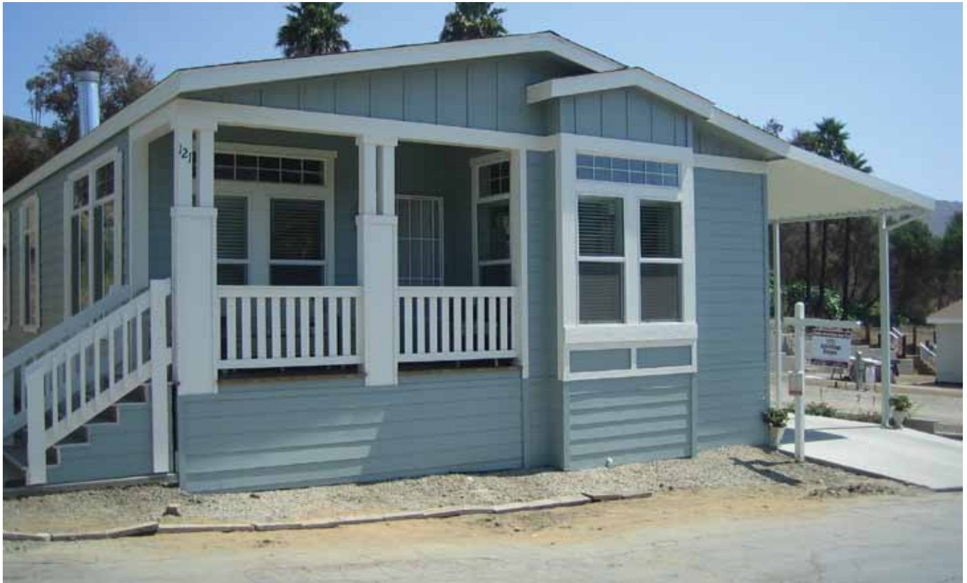
Rebuilt house in Fallbrook
